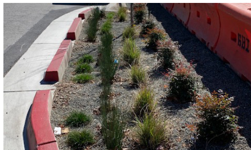
Bioswales filter pollutants
